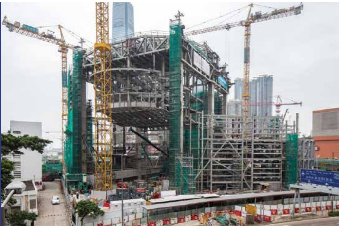
大劇院升頂後，建築結構清晰可見 The structure of the Grand Theatre is clearly visible after the steelwork is lifted to the top of building
