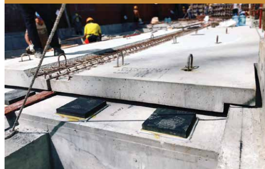
預製樓板放置在承重墊上 Precast slab sits on bearing pads
