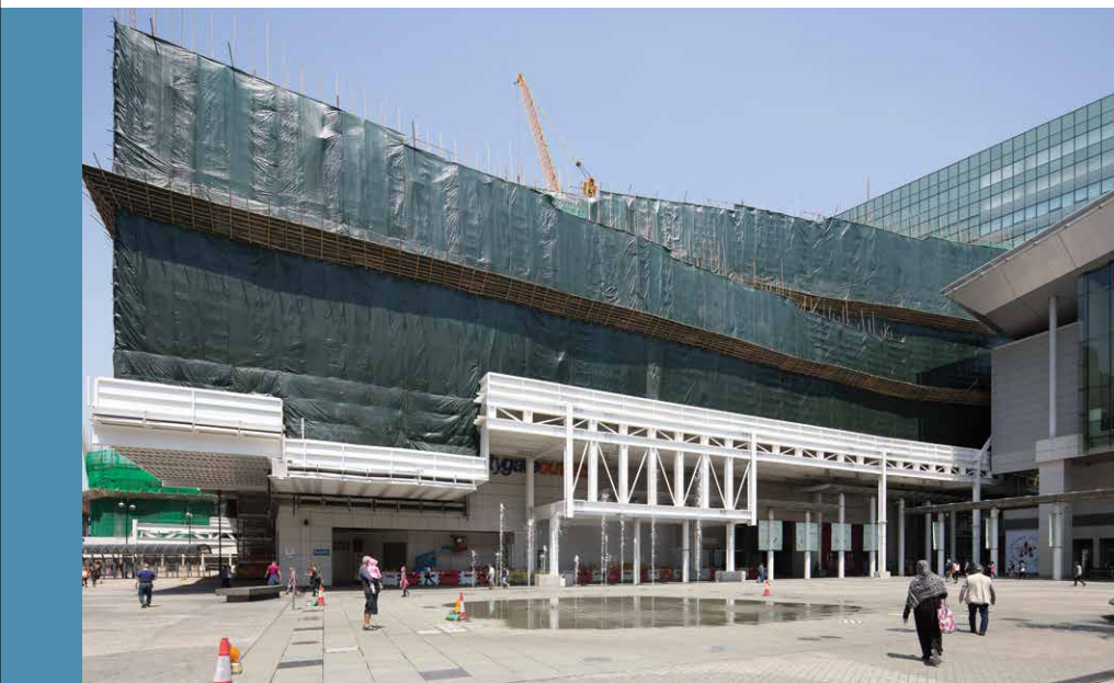
拆卸的商場範圍裝上鋼結構圍欄和保護台，以策安全 Steel fences and catch platforms are built for the demolition works to ensure safety
