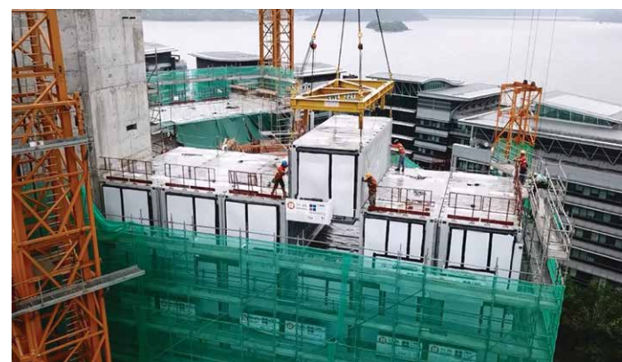
工程團隊把組件吊起並嵌入已設定的位置 Modules are lifted and fit to designated spots
