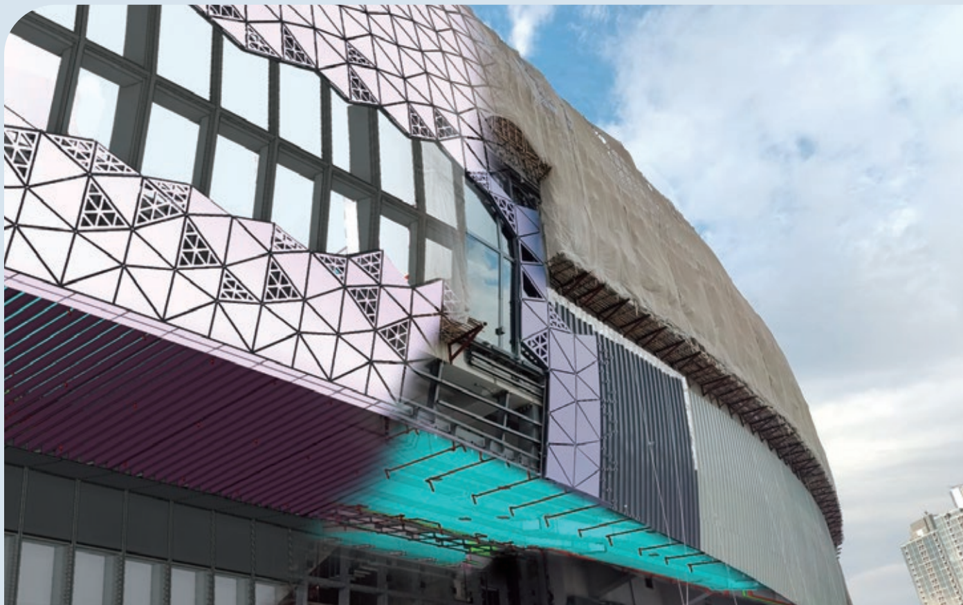
協興首次應用數位孿生建造幕牆。 Digital Twin is firstly adopted in Hip Hing to construct façade system.
