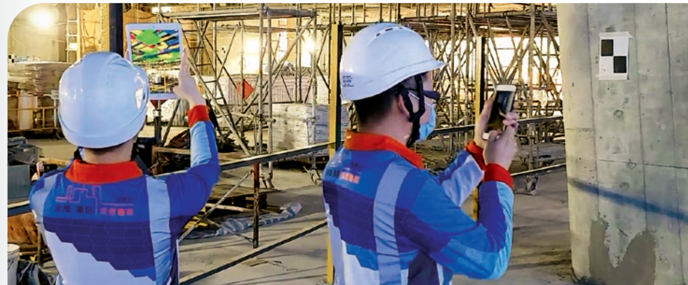
AR技術將現實及BIM模型結合，讓團隊審視施工是否與設計意圖相符。 The AR technology combines the real world and the BIM model, enabling the project teams to examine if the construction aligns with the design intent.
