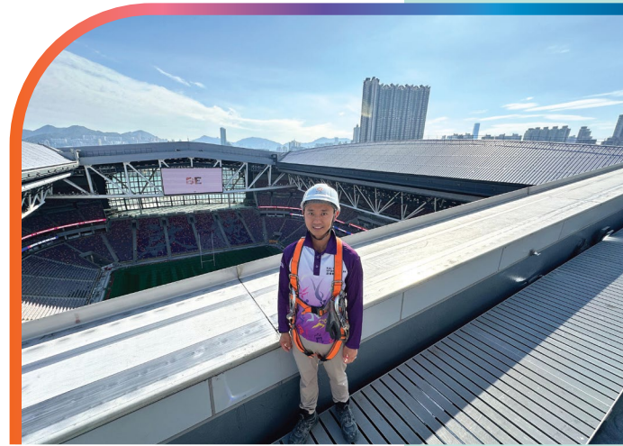
協興助理經理(建築工程)林泊光目睹工程任務完成，非常滿足。 Hip Hing Assistant Manager (Engineering) Lam Pak Kwong was very satisfied when he saw the completion of the project.
